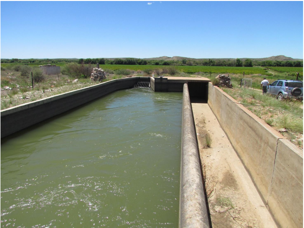
Figure 3-3: Siphon inlet to Gariep canal
